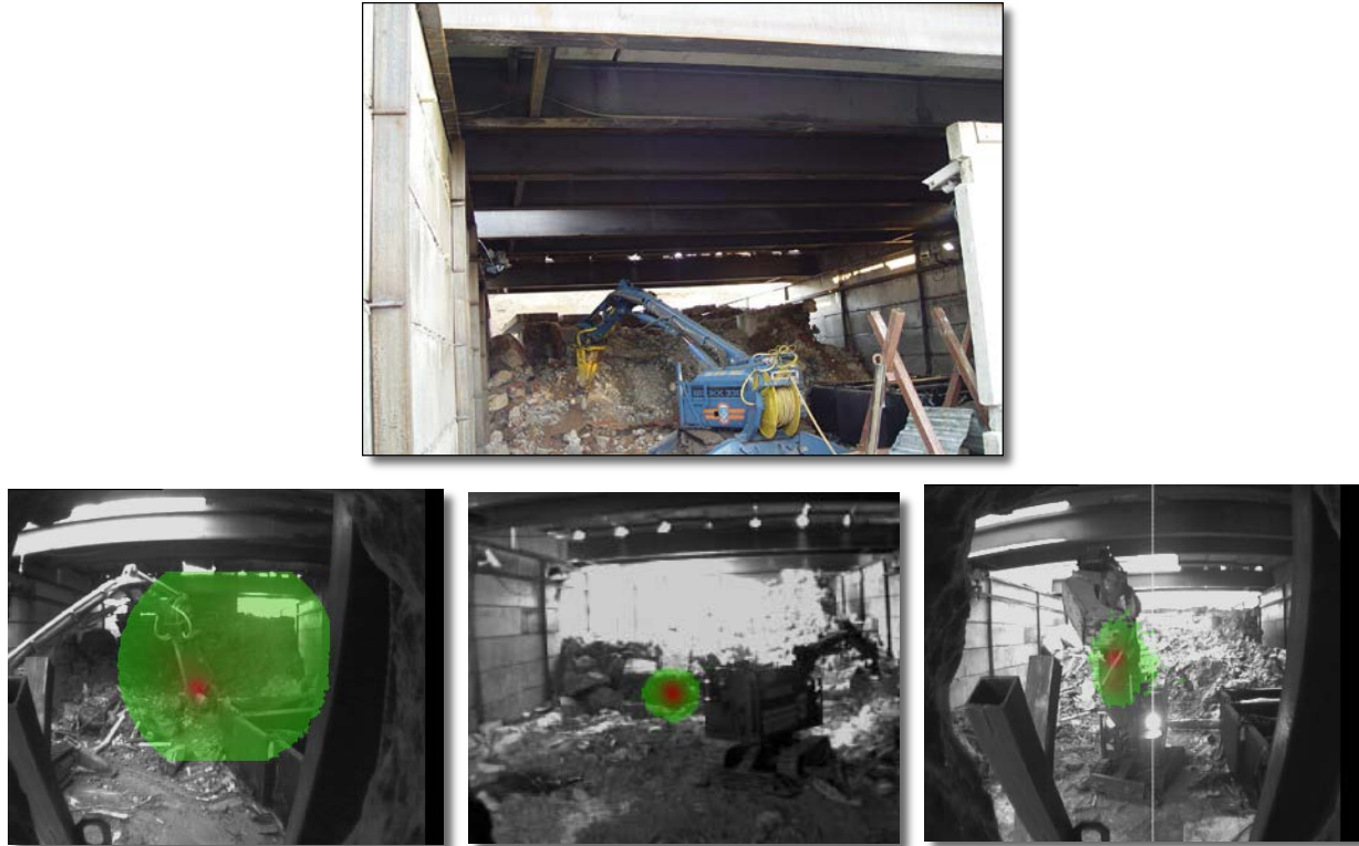
Fig. 11. Remote controlled machine is removing canisters from historical radwaste storage (above) and gamma-camera images in different moments during work (bottom row)
