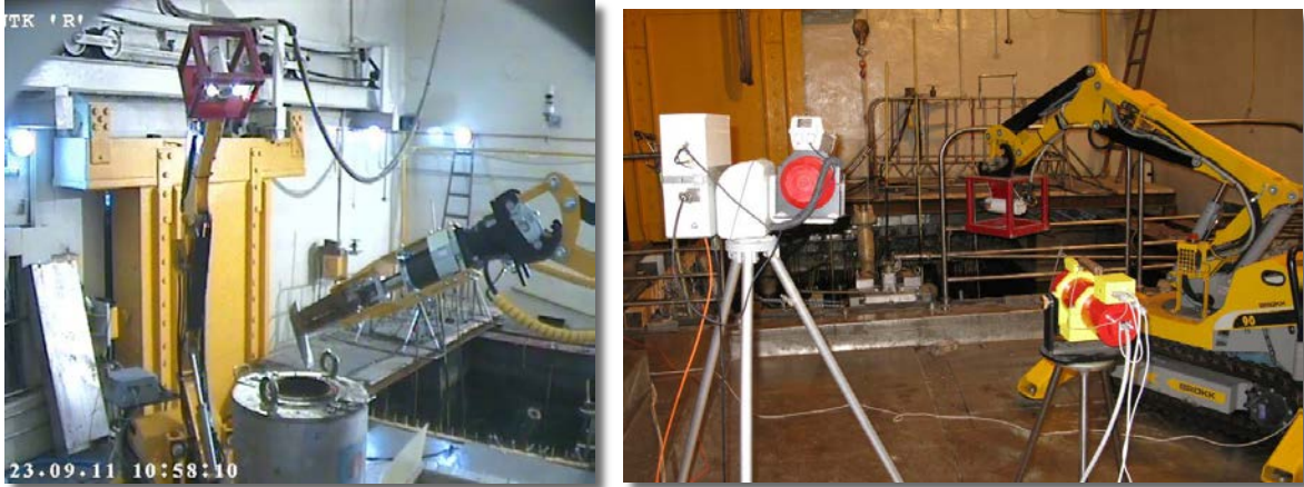
Fig. 15. Arrangement of remote controlled machine and measuring devices during operation on cutting of contaminated elements of the loop channel's part.
